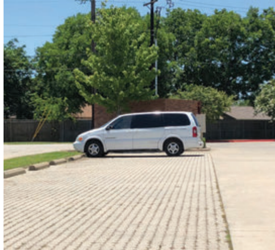
Pervious pavement in parking stalls
