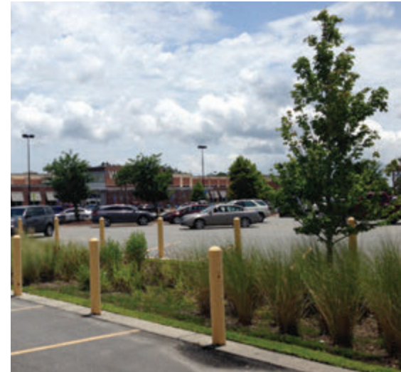
Bioswale designed into a parking lot
