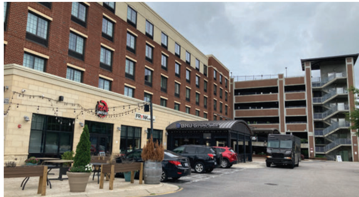
Existing parking garage in downtown
