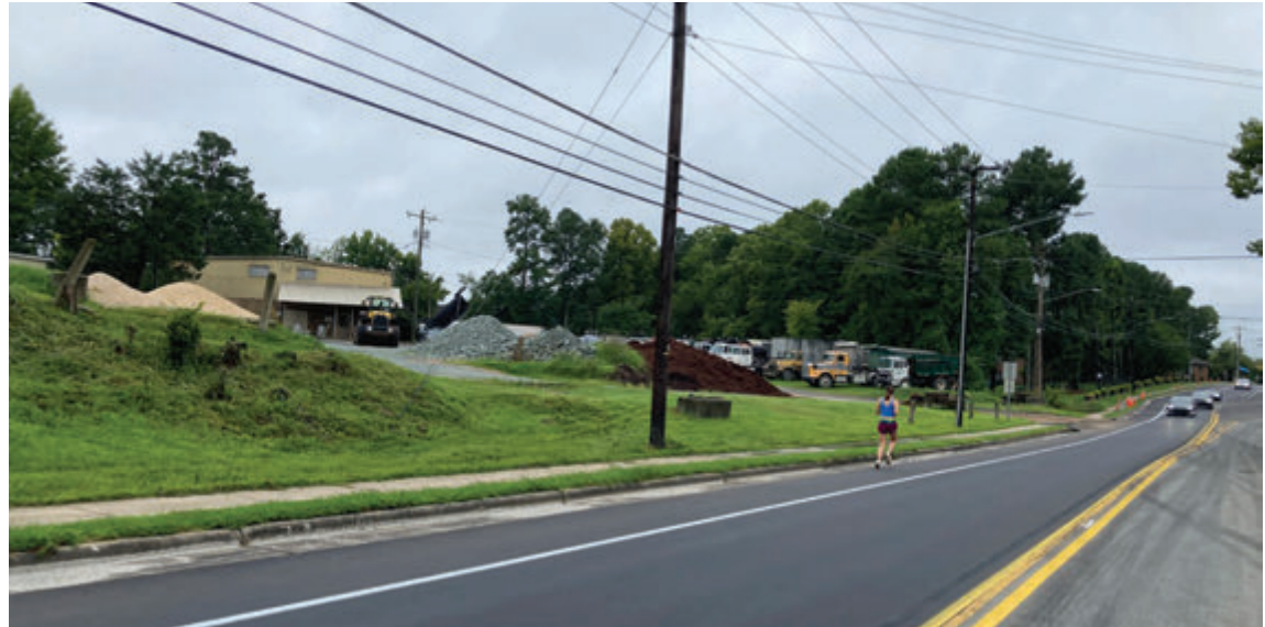
Overhead utility lines along Jones Ferry Road
