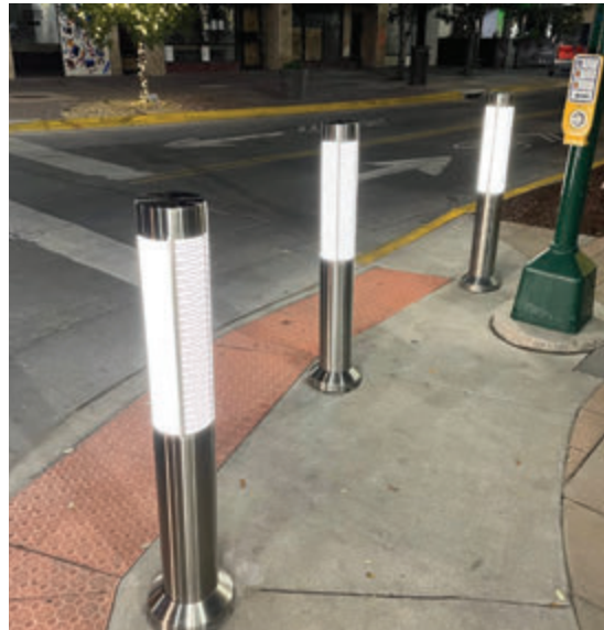
Pedestrian bollards at an intersection
