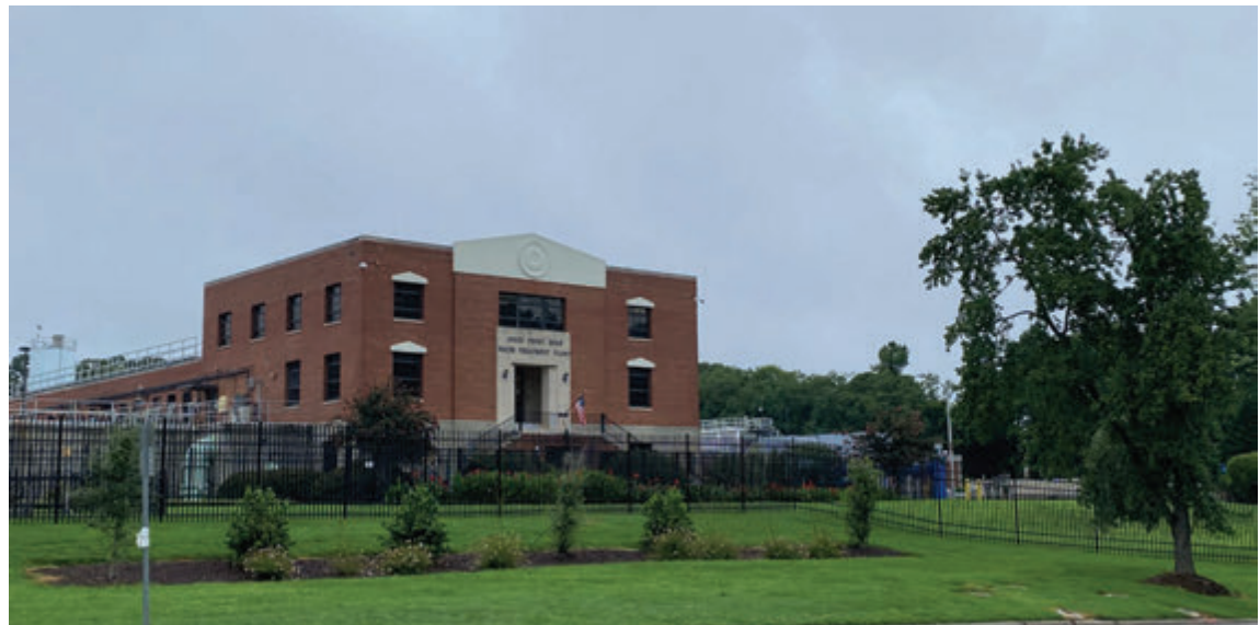
OWASA Jones Ferry Road Water Treatment Plant
