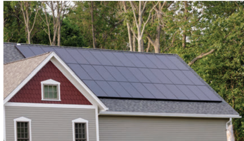
Residential scale solar application
