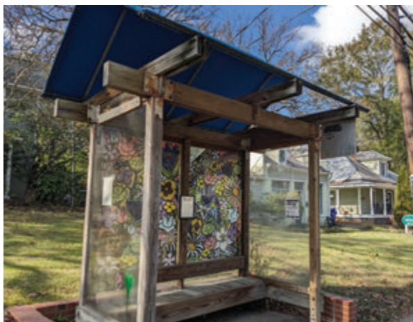
Bus shelter on North Greensboro Street
