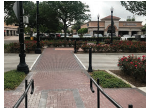
Enhanced crosswalk paving
