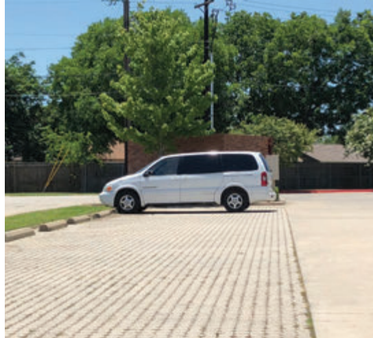
Pervious pavement in parking stalls
