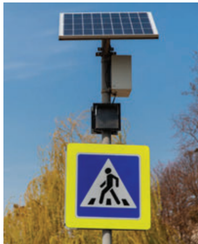
Small scale solar application
