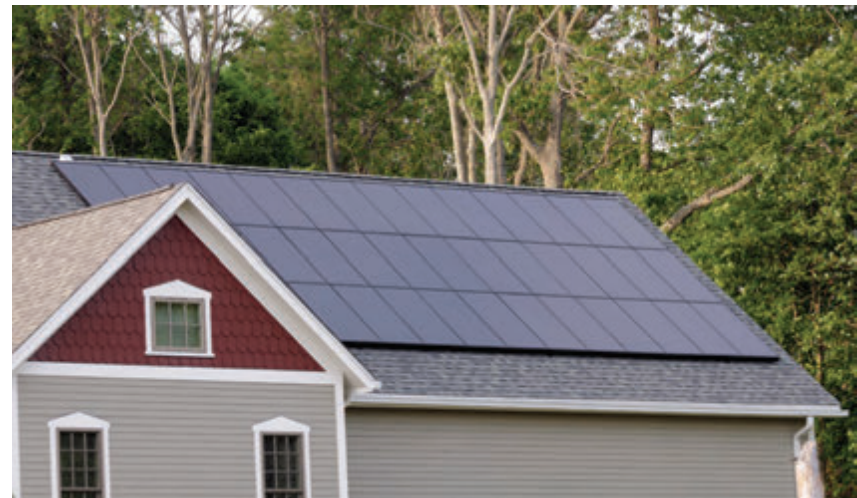
Residential scale solar application
