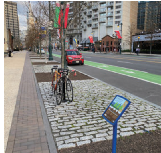
Curbside rain garden
